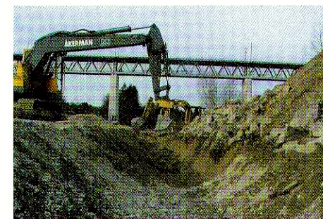
Dynamically developing bank with reverse defence system (in this case in the form of a trapeze-shaped security ditch)
