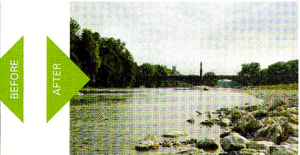
Post-restoration, the Isar is typified by gravel shorelines and banks, inlets and islands on the riverbed. It can now change and adapt with every flood. Its shoreline consists of both sloping banks and steep wash-outs and its gravel islands shift back and forth with the currents. The river's dynamism has been reactivated and a wild river landscape regained – right in the middle of the city!
