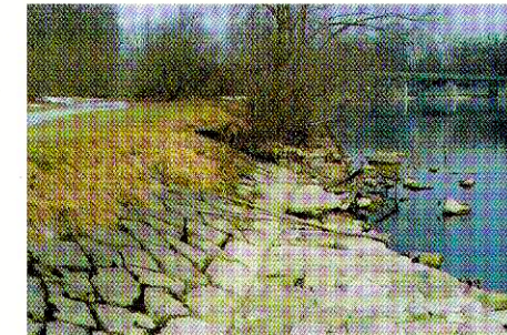
Steep, inaccessible stone banks, canal-like, monotonous shoreline prior to renaturation measures
