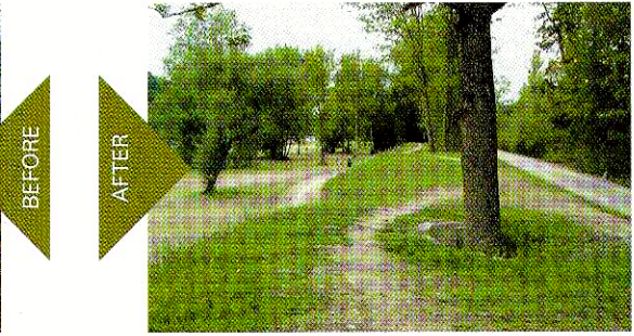
The new dykes are sufficiently high and wide. By reinforcing the dykes in front of the old embankments, the trees on the dyke crests were preserved. Flower-rich, rough pastures are developing on the new slopes.
