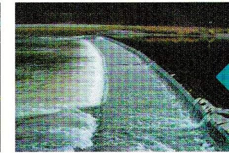
The series of cross-river sills built into the river every 200 metres prevented the straightened river from eroding away at its bed and made it impossible for the fish to embark on spawning migrations. In periods of low or medium water flow, they turned the Isar into a chain of dammed ponds.
