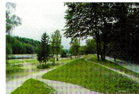
Dyke filling measures in order to preserve the existing tree population
